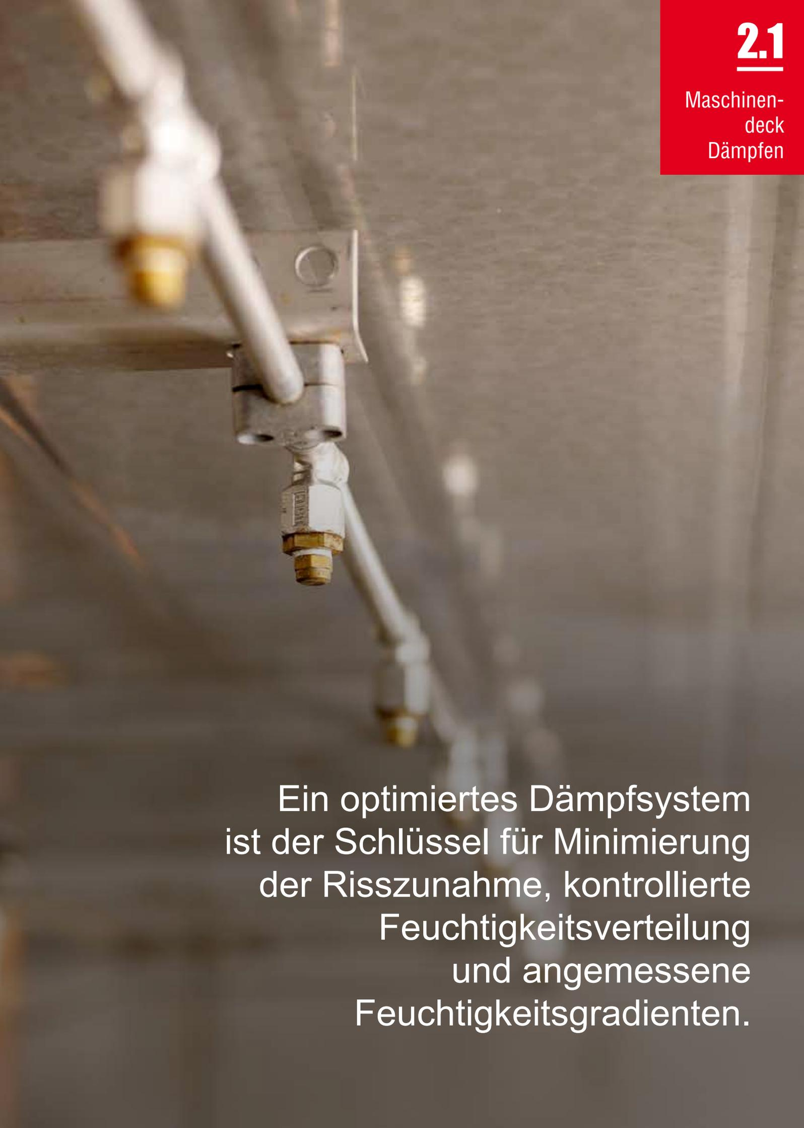
A close-up photograph of a steam nozzle assembly on a machine deck. The nozzle is made of metal and has a brass-colored tip. It is connected to a white pipe. The background is a blurred metal surface.
